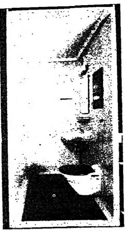
Factory-made bathroom unit, ready for shipment by lorry to a building site.
